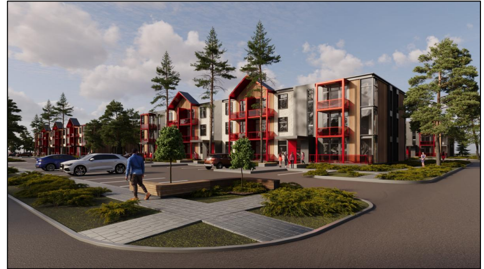
Student Union Site (New Construction, 96 Units)
