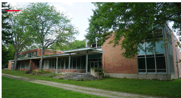
With plans to demolish the site, Columbus-based Windsor Companies purchased the Antioch
