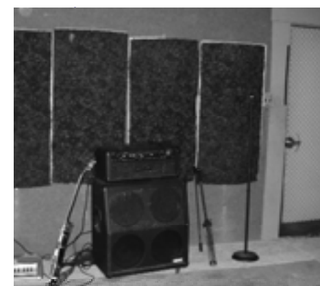
Students applied soundproofing material such as carpet, foam and egg cartons to the walls and ceiling to sound-proof the recording studio.
